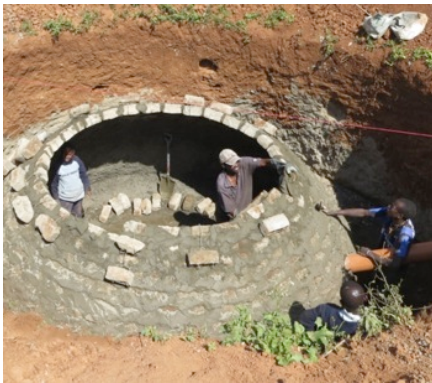
Installation of the biogas digester
