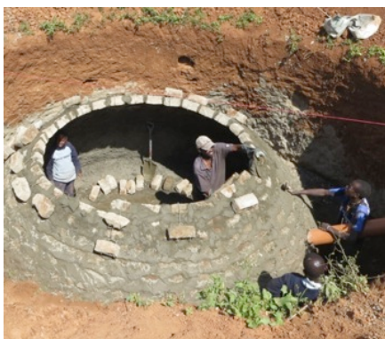
Installation of the biogas digester
