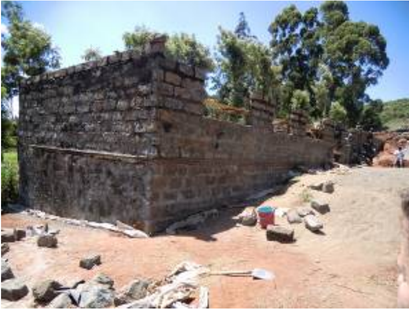
Foundation and wall
