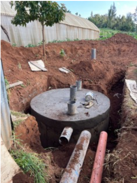
Biodigester is almost finished
